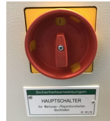
Fig. 16: Example: Main switch for switching the lift on and off
